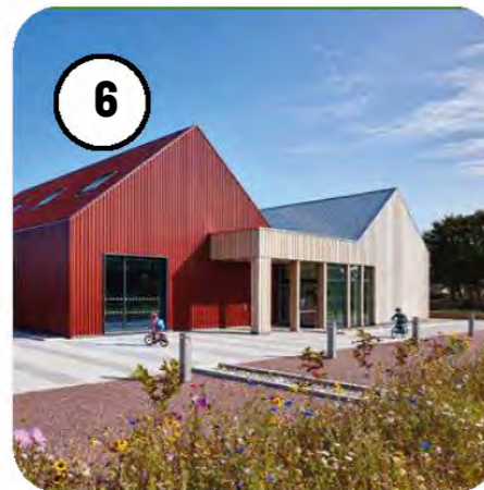
6 Highly visible edge plots. Elevations offer opportunities to integrate the development into the park and provide identity.
